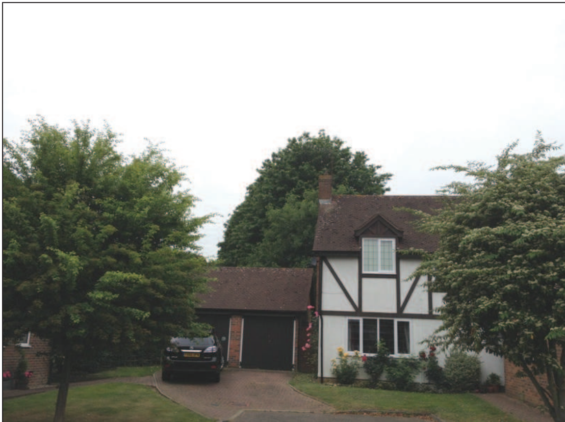
Figure 3: The view of the Oaks from outside 7 Deerings Drive
