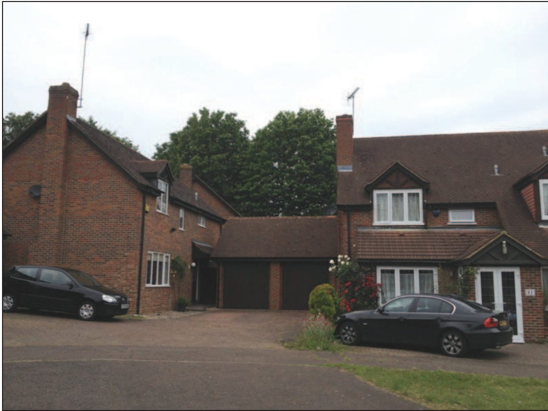
Figure 2: The view of the Oaks from outside 21 Deerings Drive
